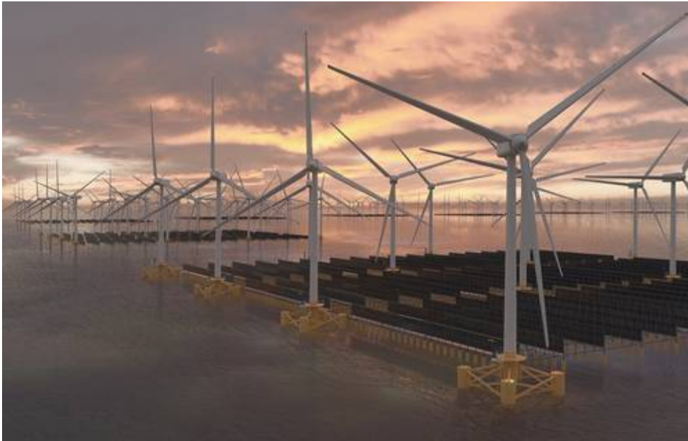
Figure 11. Offshore floating platform integrating solar photovoltaic panels with a wind turbine for hybrid energy generation ( “Tadek Ocean Engineering Expands UK Office,” n.d. ).
