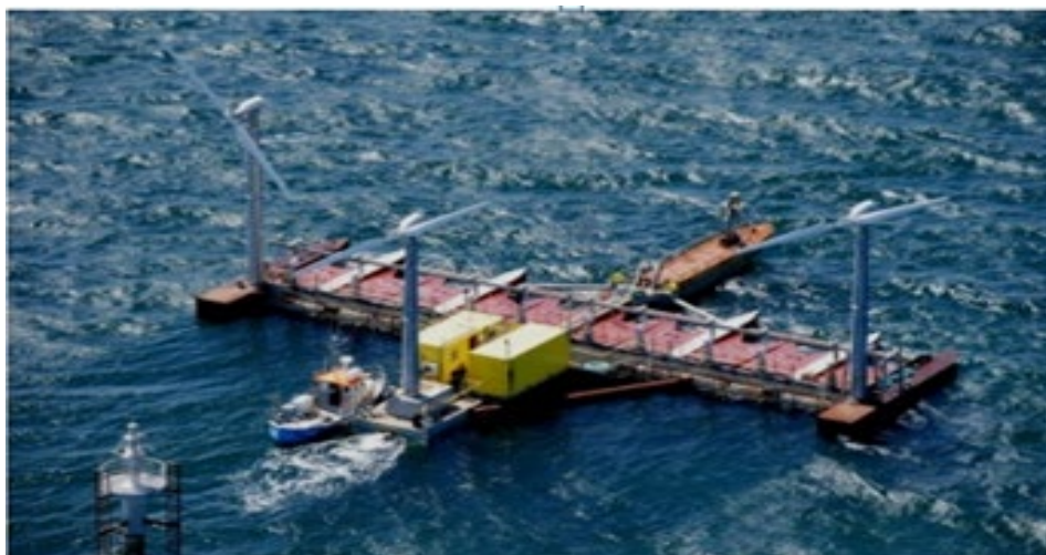
Figure 8. Poseidon hybrid floating system combining wind turbines and wave energy converters (Tomey-Bozo et al., 2015).
