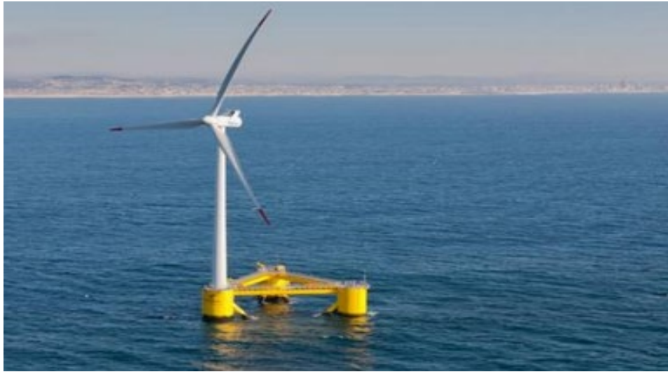
Figure 9. Wind Float semi-submersible floating wind turbine and wave converter.
