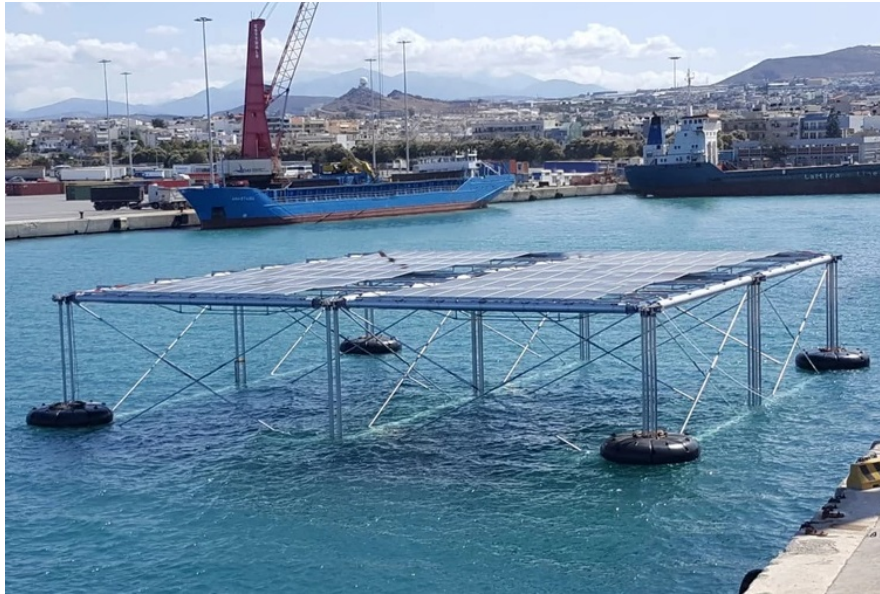
Figure 13. 80-kW floating energy system created by Sinn Power, located in Heraklion, Greece.
