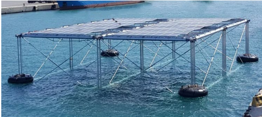
Figure 10. Offshore floating platform integrating solar PV panels with wave-energy converters (Bellini, 2021a).
