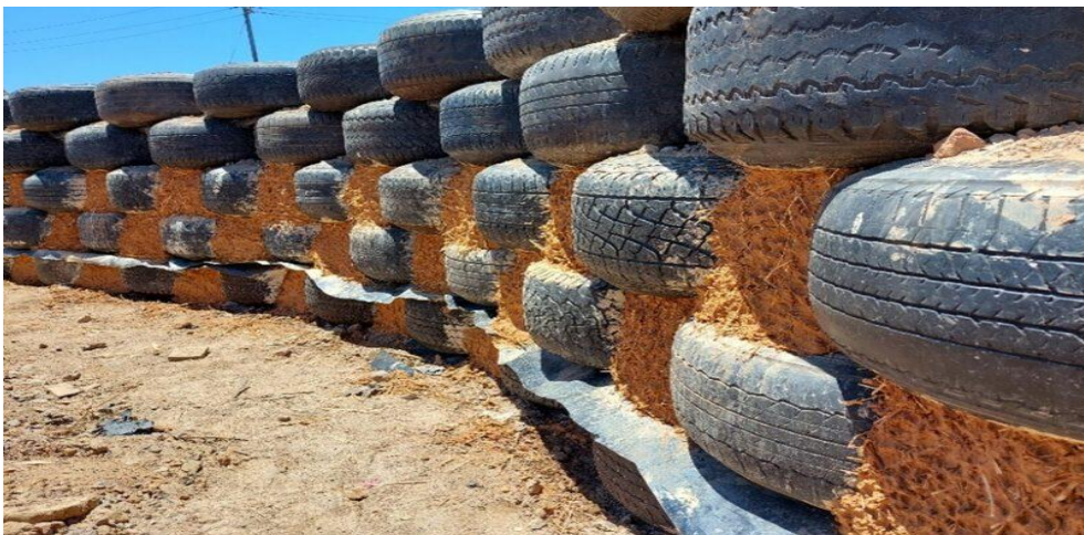
Figure 5. Passive design of the tyre walls illustrates the use of compacted tyre construction to support thermal mass.
